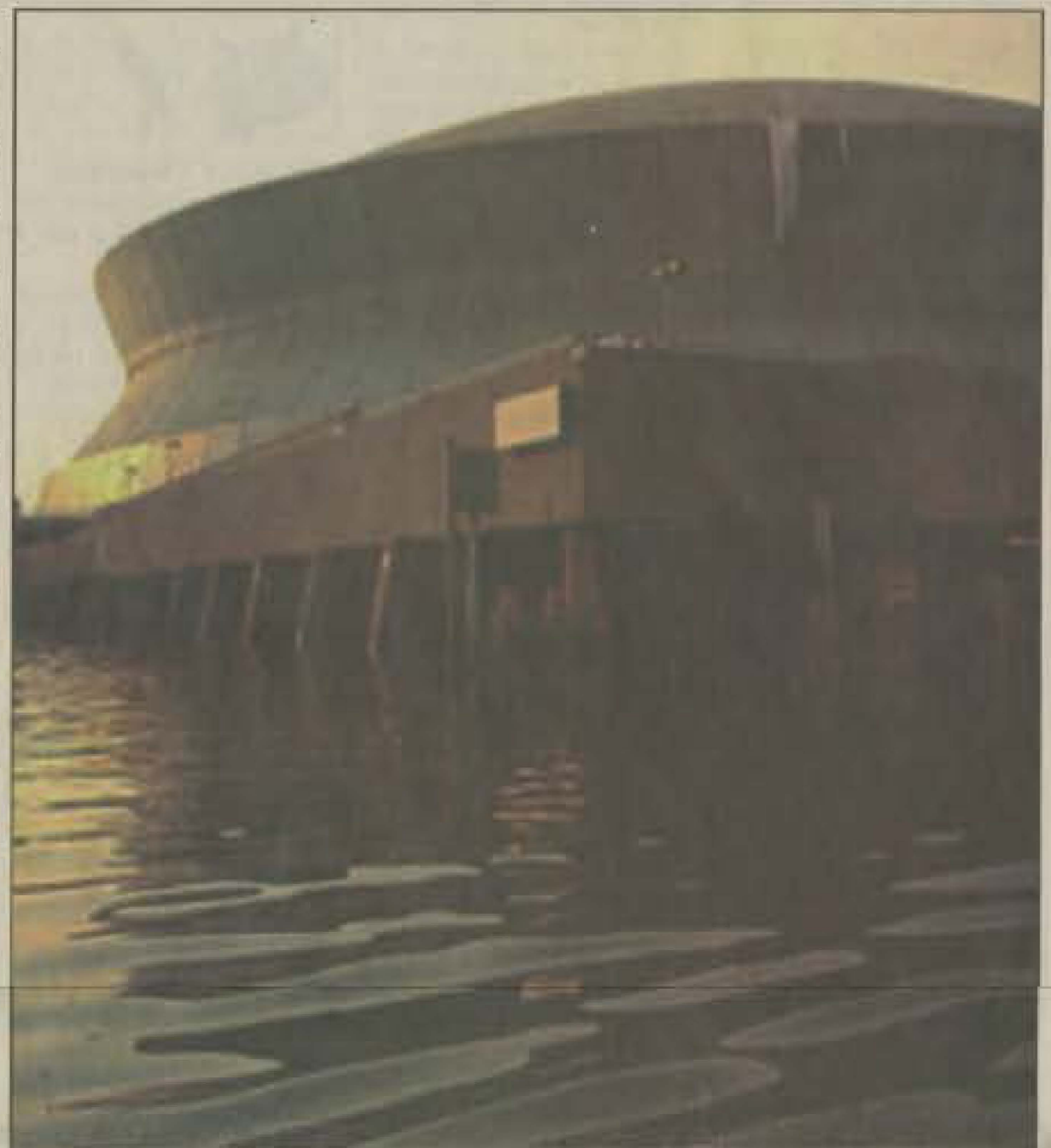
Louisiana's governor's office says the Superdome, which temporarily sheltered evacuees, may be torn down due to damage by the flood. Seen here, the Superdome is under several feet of water.
