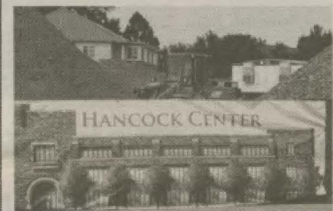
RYAN HUTTON / THE CIRCLE Construction on the Hancock Center has displaced some faculty parking.
