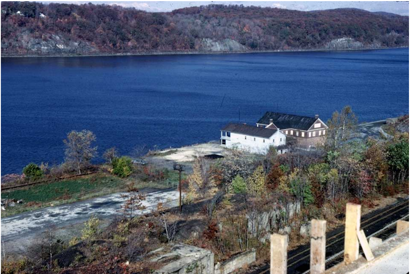
View of boathouse row before construction of the Martin Boathouse, taken from one of the unfinished upper floors of the Leo Dormitory. The California and Cornell boathouses were used by the high schools, and Dutton Lumber began shrinking its supply of aging lumber.
