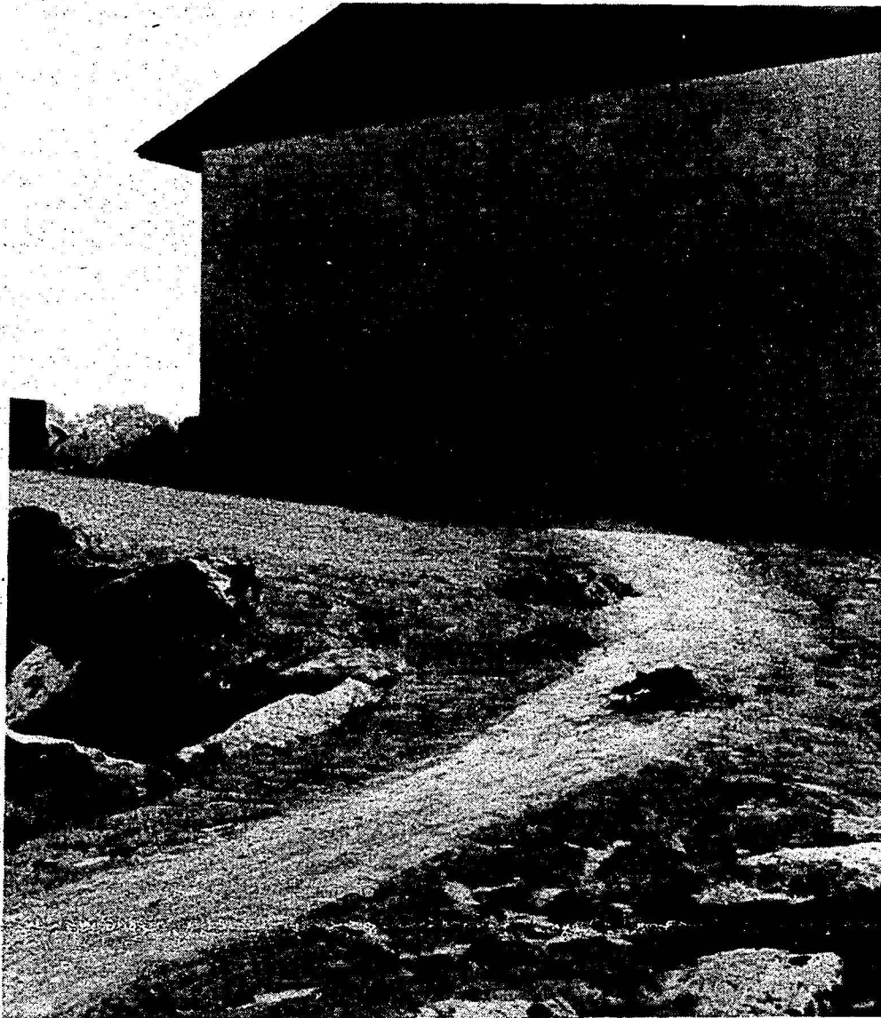
The ramp system at the new townhouses has been the target of criticism by Linda Glass, a Marist student who uses a wheelchair and wants to live in the townhouses.
