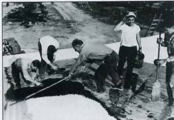
Marist Brothers work on the roof of Donnelly Hall.
