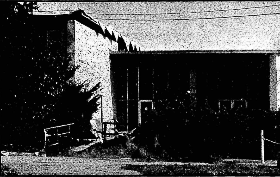
Work on the new patio for Donnelly Hall is scheduled to be completed this week.
