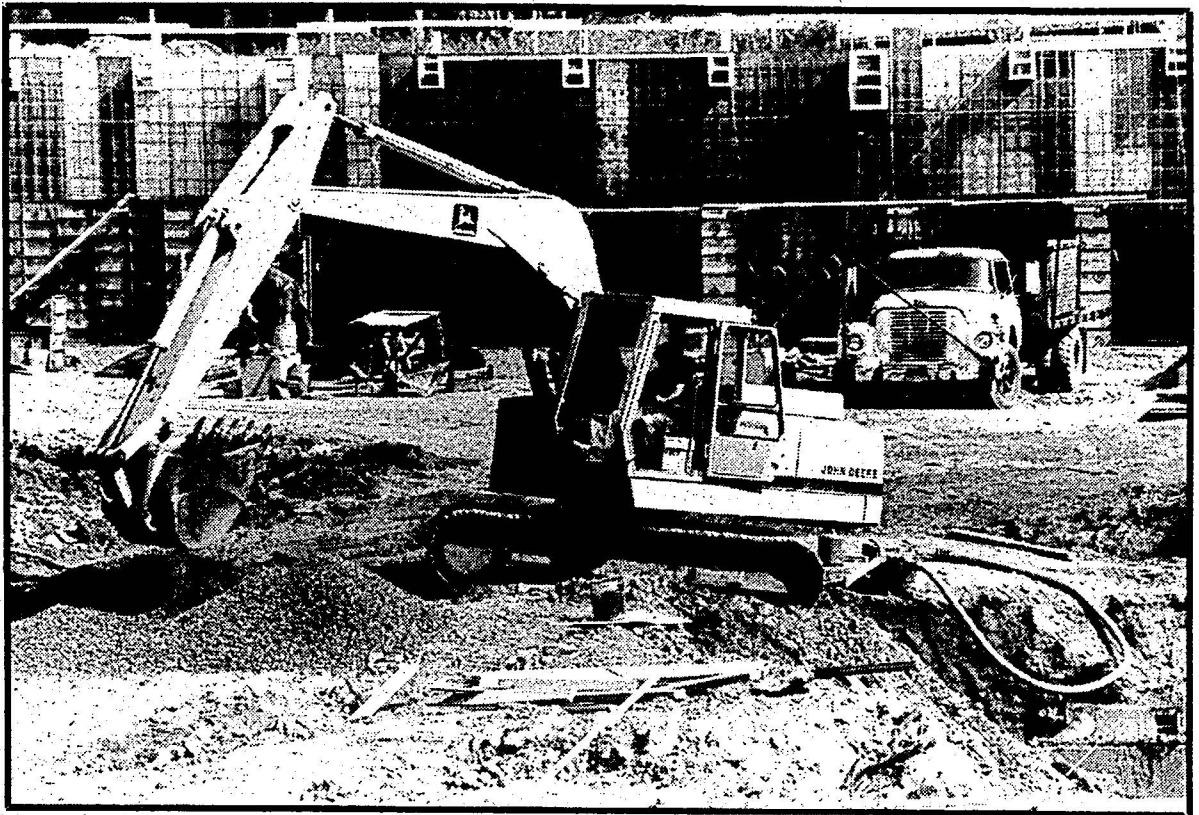
Construction continues on the Lowell Thomas Communications Center. The center's tentative completion date is now January 1987. (photo by Bryan Mullen)
