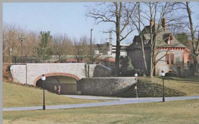
Pedestrian walkway under Route 9
