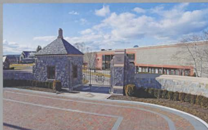
New main gate
